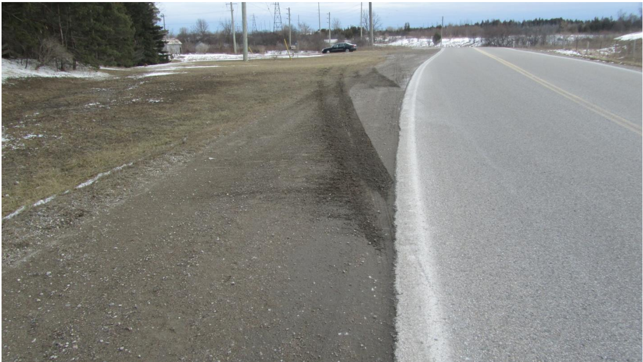
Figure 44: View, looking south, at the tire marks of the southbound vehicle as it enters the east shoulder and roadside.
