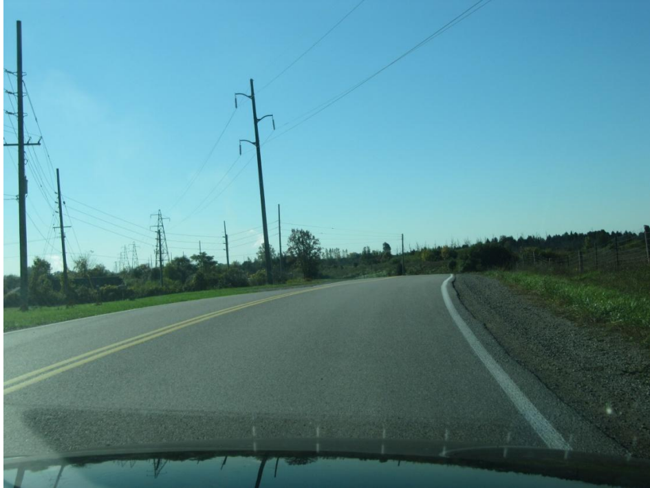
Figure 3: View of the line of sight of a typical driver travelling southbound in a passenger car while passing through the north curve of the S-curve. The view of the road ahead is limited.
