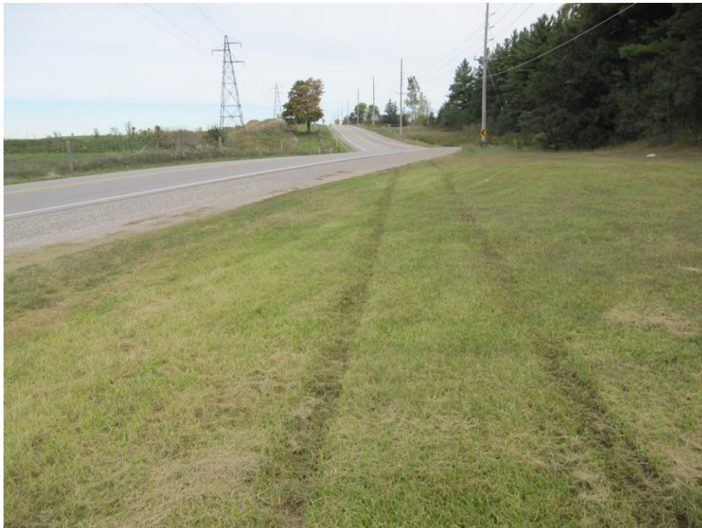
Figure 25: View, looking north, at the tire marks of a southbound vehicle which exited the roadway a short distance south of the north curve.
