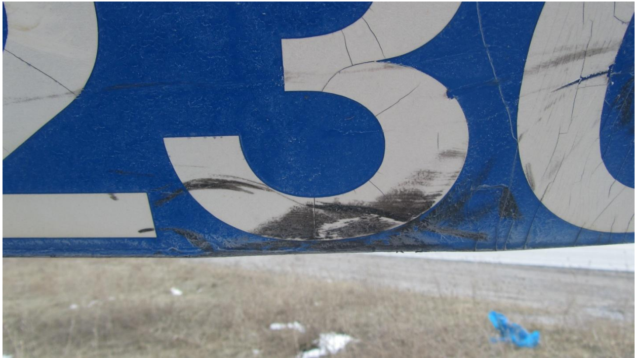
Figure 50: Close-up view of the black transfer on the address marker caused by contact by the southbound vehicle.
