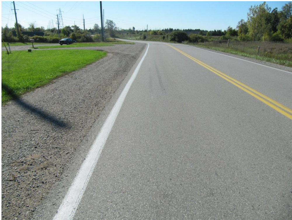
Figure 5: View, looking south, toward the east roadside between the two curves.
