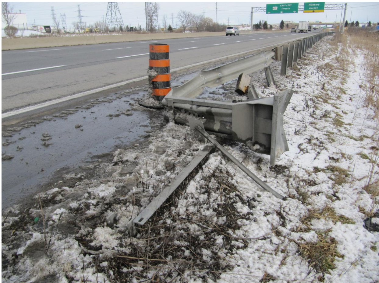
Figure 3: View showing how the ET-Plus terminal has rotated ninety degrees with respect to the length of the rail. Clearly, if any additional energy had to be dissipated it would not take place via the passage of the rail through the throat of the terminal.
