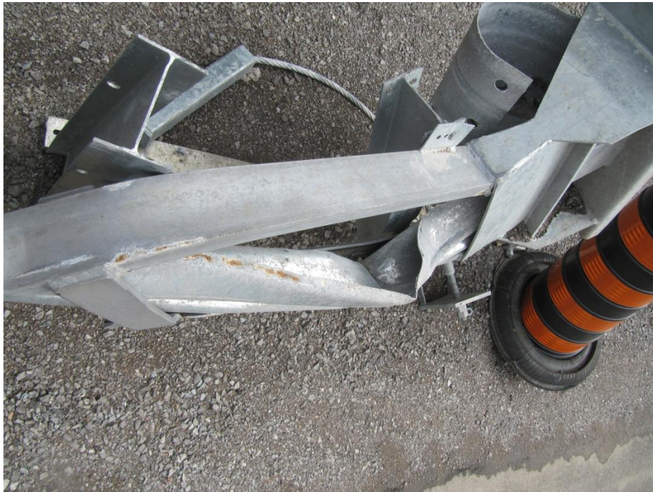
Figure 27: Top view showing that the guard rail is buckled within the channel.
