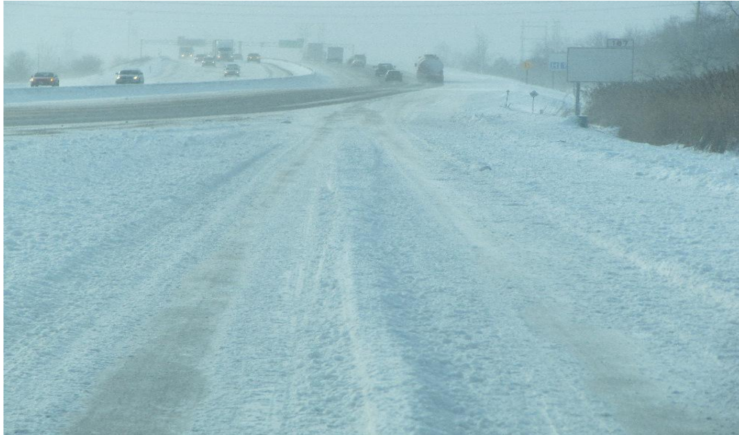
Figure 1: Highbury Ave entrance ramp onto Hwy 401 in London, Ontario on January 25, 2014. Unplowed ramps and shoulders along the 400 series of highways was one of the winter road maintenance problems identified in the Auditor General's report of April, 2015.
