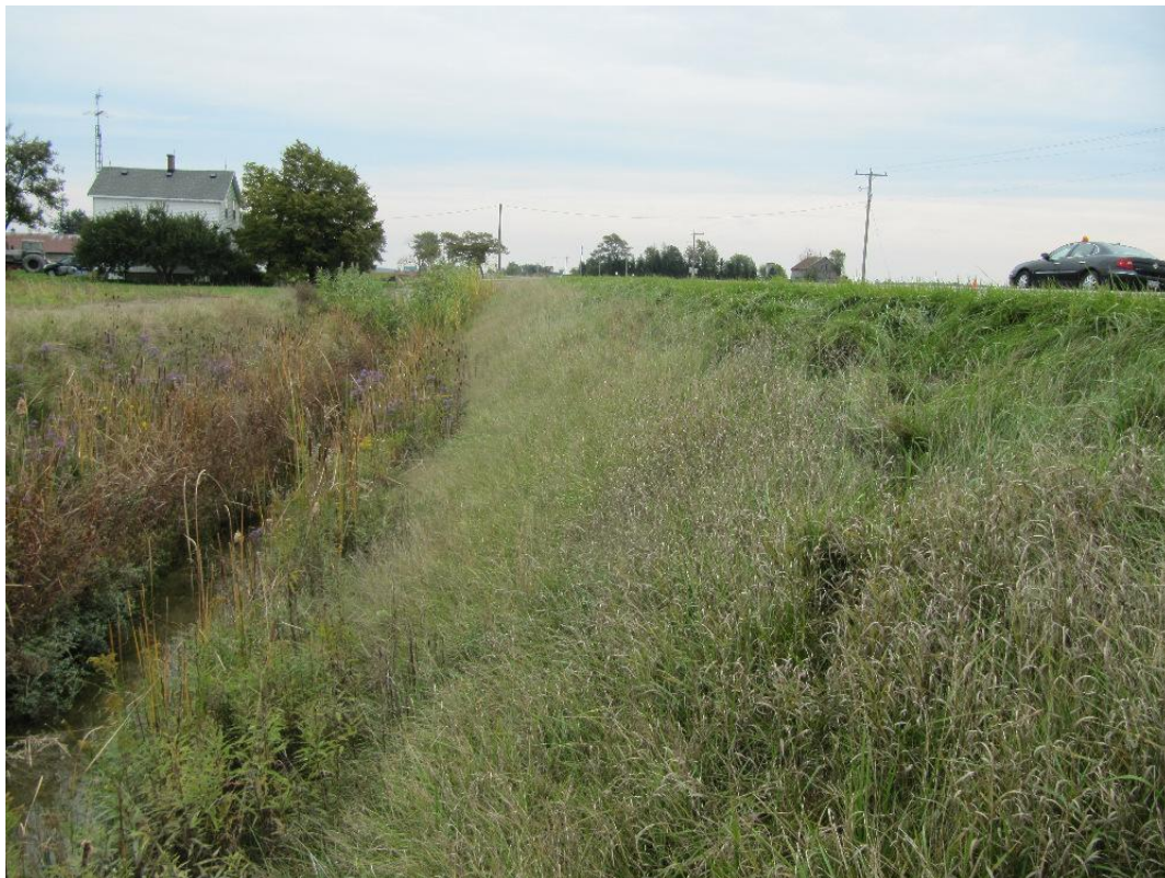
Figure 6: Eastward view of depth of north ditch and steepness of its embankment, on the opposite side of where the police cruiser came to rest.
