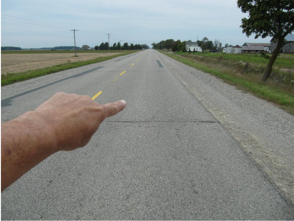
Figure 15: View, looking west, with investigator's finger pointing to the location where the cruiser's yaw marks first became visible in the westbound lane.
