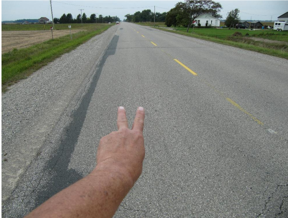
Figure 14: Westward view with investigator's fingers pointing out the two yaw marks in the eastbound lane indicating that the cruiser was rotating clockwise at this location.
