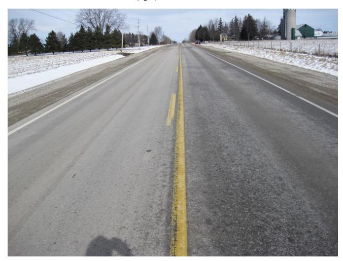
Gouges at the west edge of the southbound lane indicate that the Avalanche crossed the road centre-line and that the driver of the Tanker Truck likely steered to the right in an attempt to avoid the collision.
