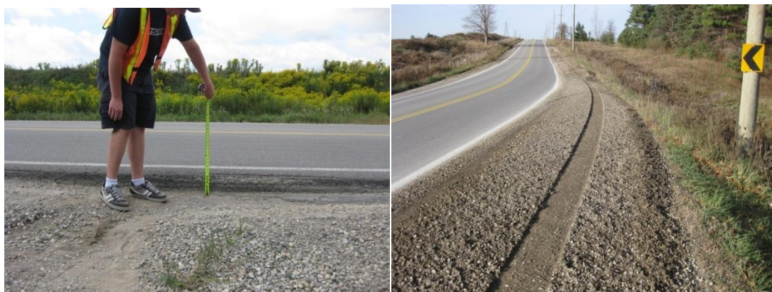
Figure 3: Drop-off on Clarke, September, 2009 (left) and deposit of fresh gravel in November, 2009 (right)
