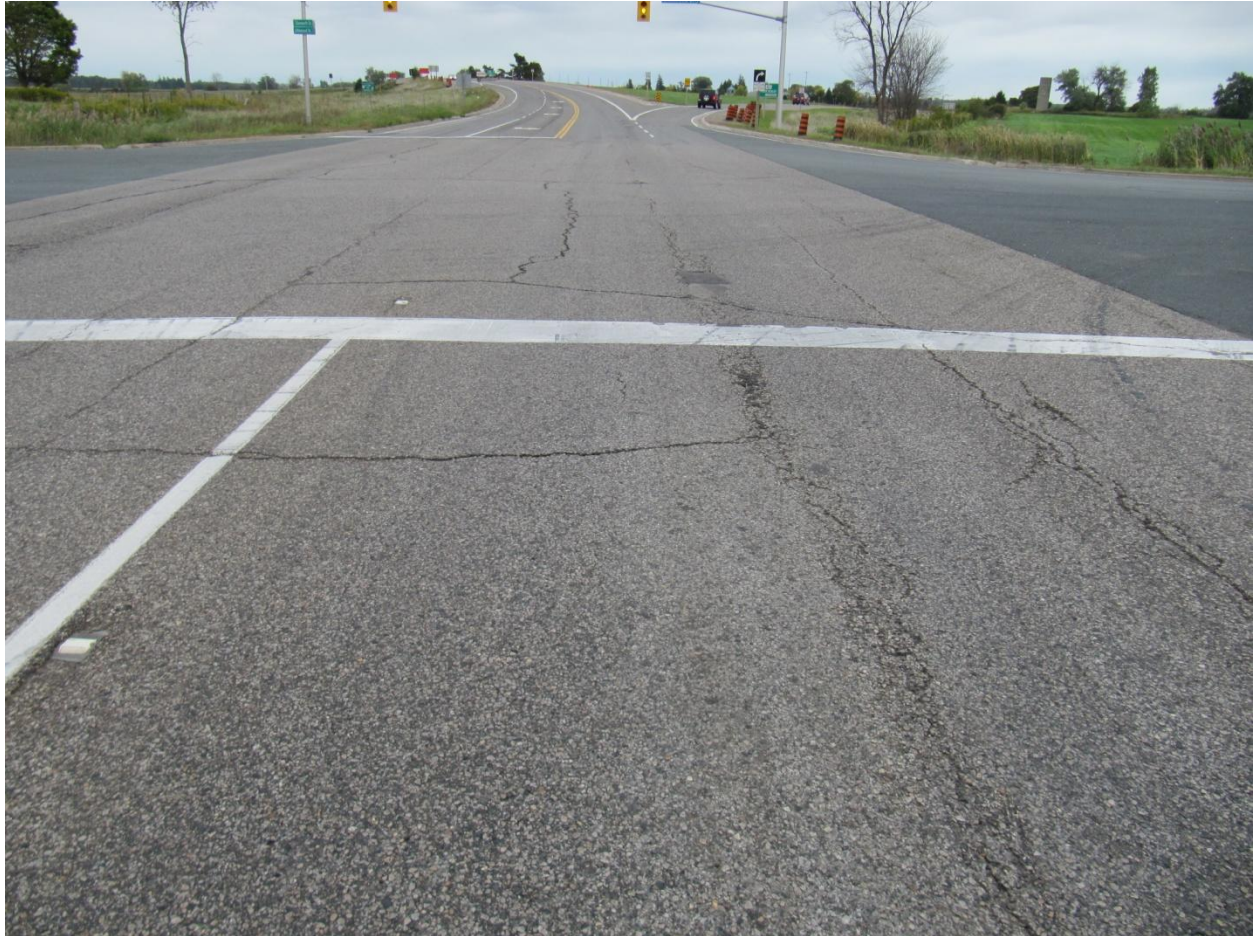
2 - View looking south at north edge of intersection with Glanworth Drive
