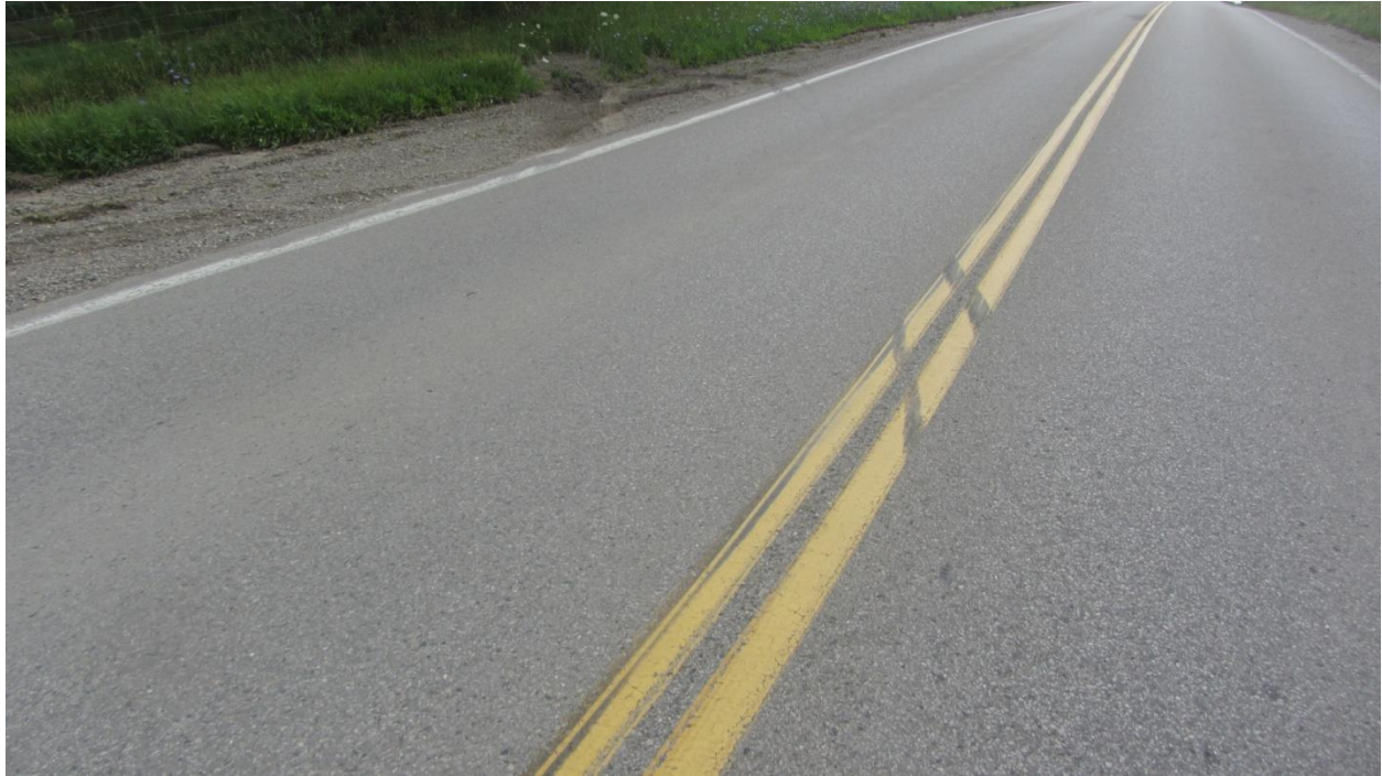
Figure 41: View looking northwest at the black yaw marks on the centre line and the tire marks on the west shoulder in the background where the northbound vehicle came to rest.
