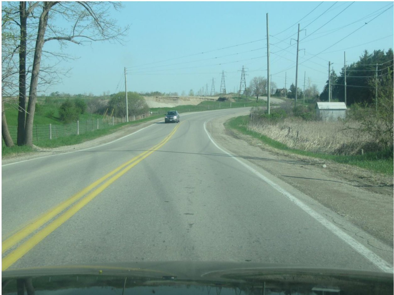
Figure 37: View looking north taken from the Gorski Consulting dash camera at approximately 1410 hours of June 21, 2014. This is upon approach to the south portion of the S-curve.
