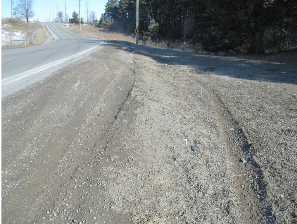
Figure 20: View looking north along the yaw marks located on the east roadside.
