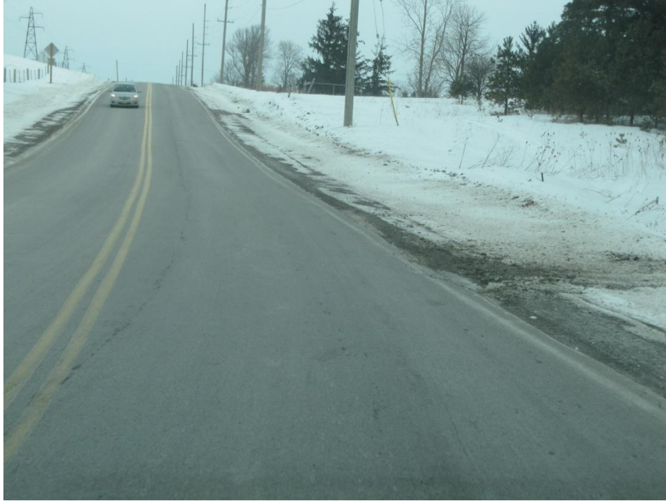
Figure 9: View, looking north at the north end of the north curve on March 4th, 2014, showing the road conditions.
