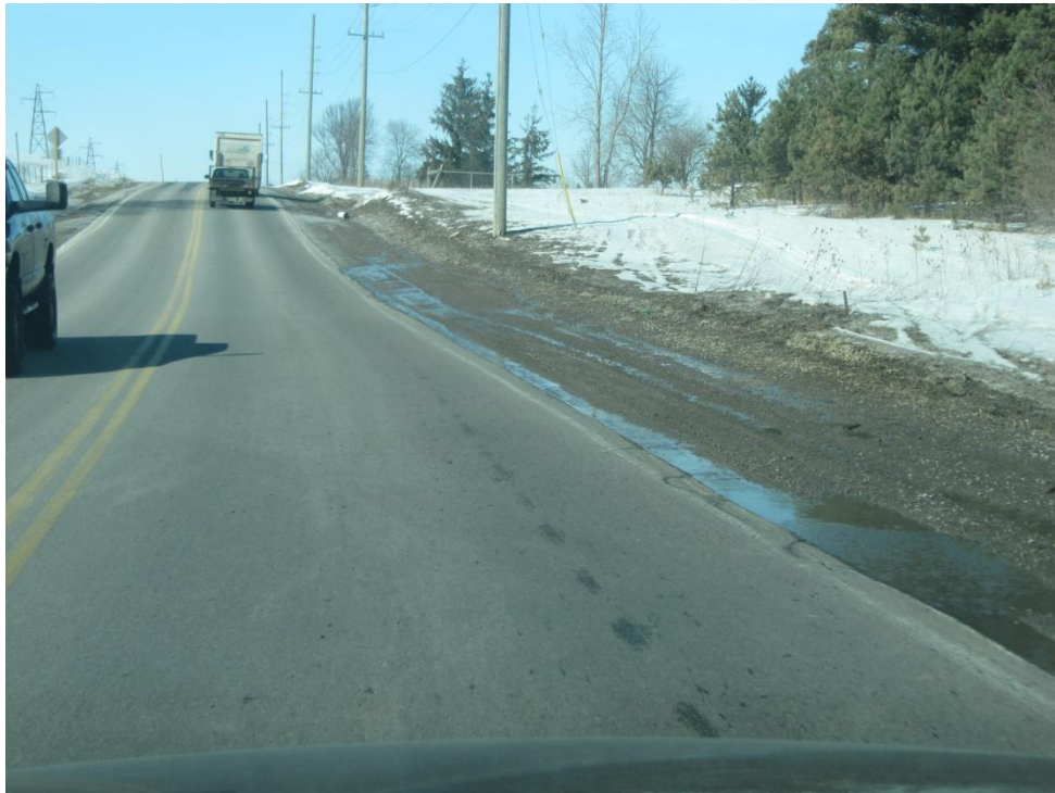
Figure 10: View, looking north at the north end of the north curve on March 7th, 2014, showing the road conditions.
