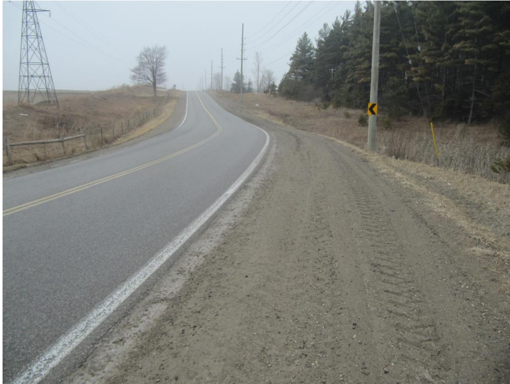
Figure 23: Collision that was documented on April 4th, 2014. This is a view looking north along the east shoulder at the north curve. Just past the utility pole a northbound vehicle travelled down the embankment and collided with the ground below.
