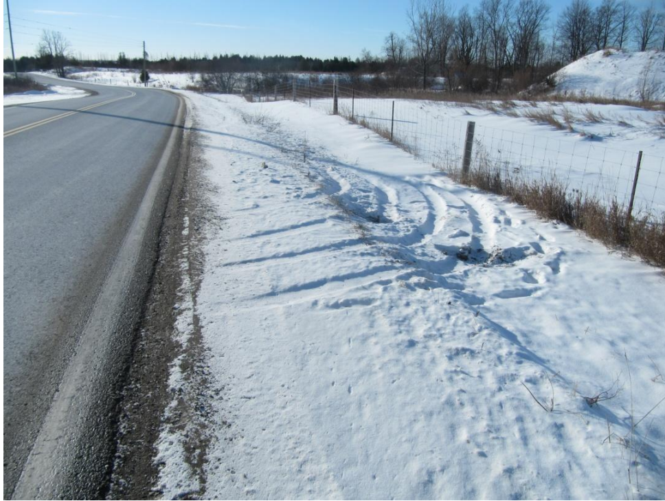
Figure 5: Incident documented on January 21st, 2014. This is a view of the evidence of a loss-of-control incident whereby a northbound vehicle slid into the west roadside. It is conceivable that his action occurred because of an impact with another vehicle on the road however the lack of further information from the police data makes it not possible to draw a conclusion one way or the other.
