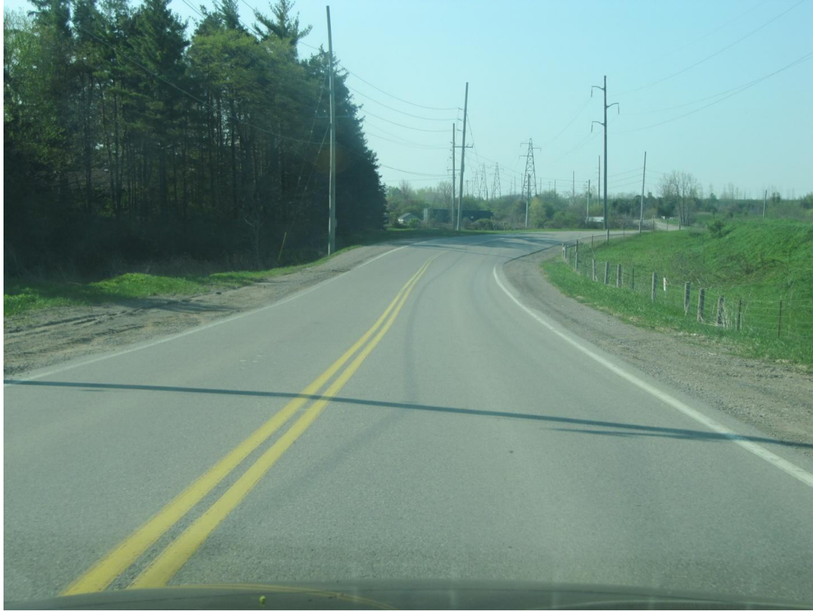
Figure 38: View looking south while approaching the north curve of the S-curve.
