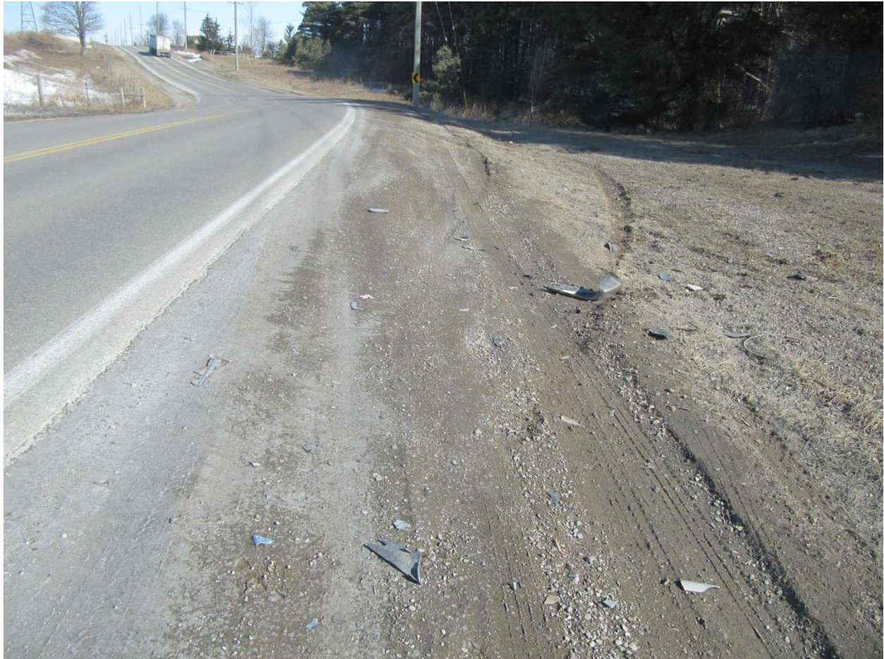
Figure 19: Collision documented by Gorski Consulting on March 18th, 2014 this is a view looking north along the east roadside. Loss-of-control yaw marks can be seen in the grass of the roadside and on the gravel shoulder in the foreground. For official purposes the evidence has been reported as caused by a northbound vehicle. However there is some doubt about that conclusion. Vehicle parts can be seen strewn around the vicinity of the tire marks indicating there was a collision but no further conclusions can be drawn.
