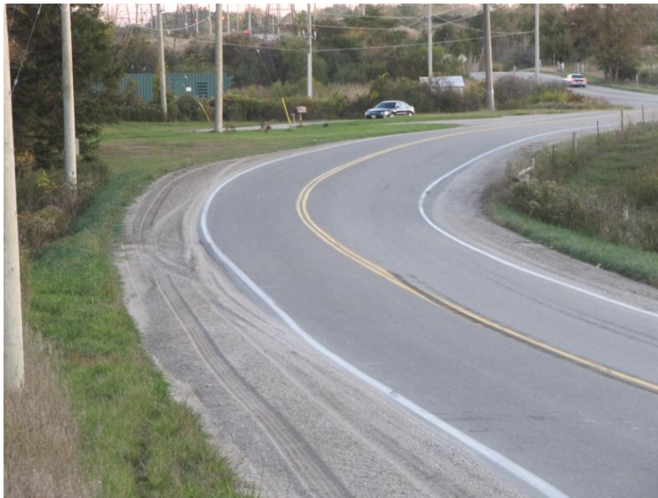
Figure 1: View, looking south, of the S-Curve on Clarke Road on October 11, 2013.
