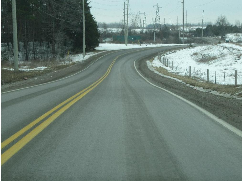
Figure 1: View, looking southbound at the S-Curve of Clarke Road north of Fanshawe Park Road in London, Ontario, showing the horizontal and vertical alignments of the road.
