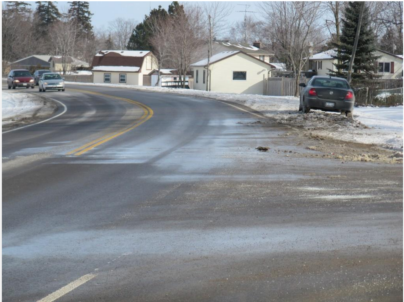
View looking north on Glanworth Curve Showing Moisture on Northbound Lane at Location Where Fleeing Vehicle Left the Roadway
