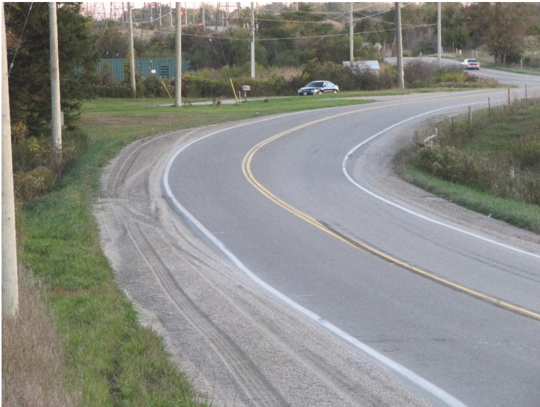
Figure 1: View looking south at the S-curve of Clarke Road north of Fanshawe Park Road in London, Ontario on October 11, 2013. This is the "Laboratory" where a number research studies have been conducted at Gorski Consulting.
