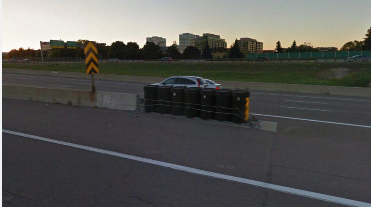
View of unusual energy attenuation device installed at the end of the New Jersey barrier which was likely struck by the bus and caused the rollover.
