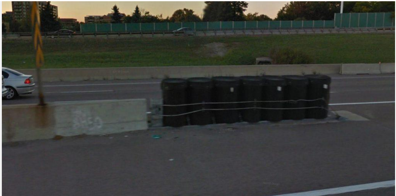
Side view of the energy attenuation device. A change in the shade of the concrete suggests it had been damaged in a previous incident.
