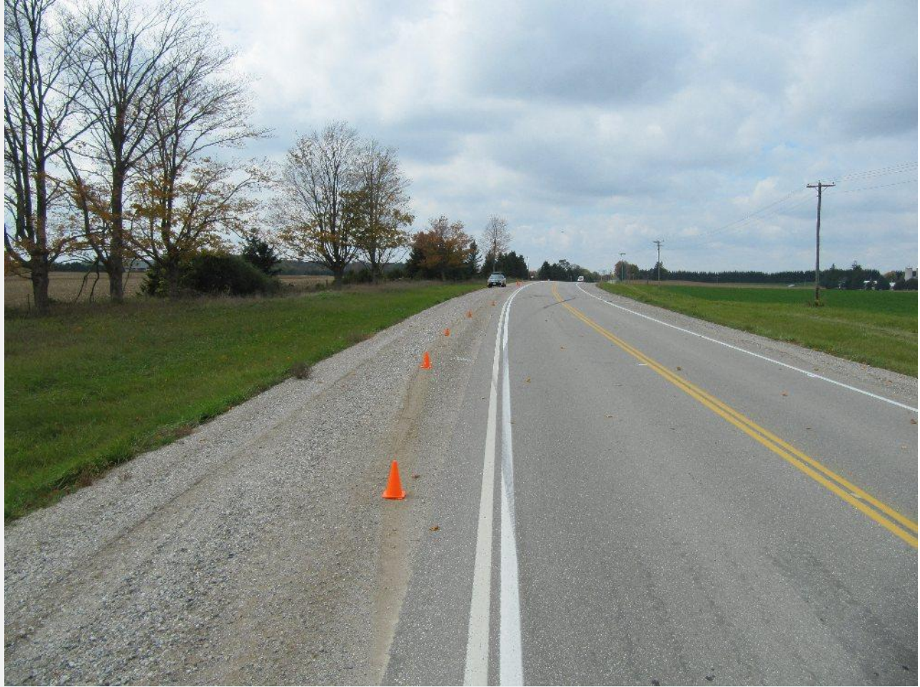
View, looking west along Road 88. The orange cones show the path of a tire mark on the south shoulder where the westbound vehicle entered and then returned to the road where the impact occurred.
