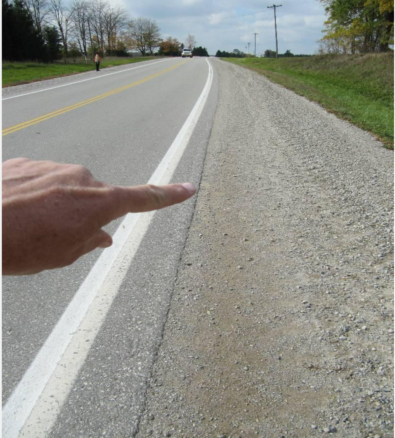
View, looking west, along Road 88. The finger is pointing to a tire mark on the right (north) shoulder where the vehicle initially left the road surface.
